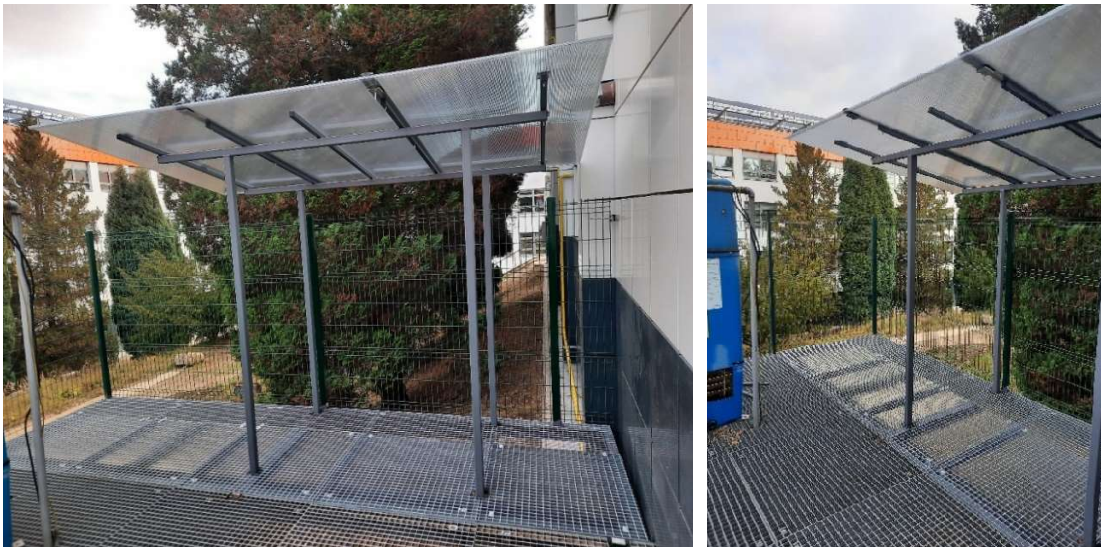
Fig. 8.7 The implemented platform with a shelter prepared for the installation of a small pyrolysis reactor.
