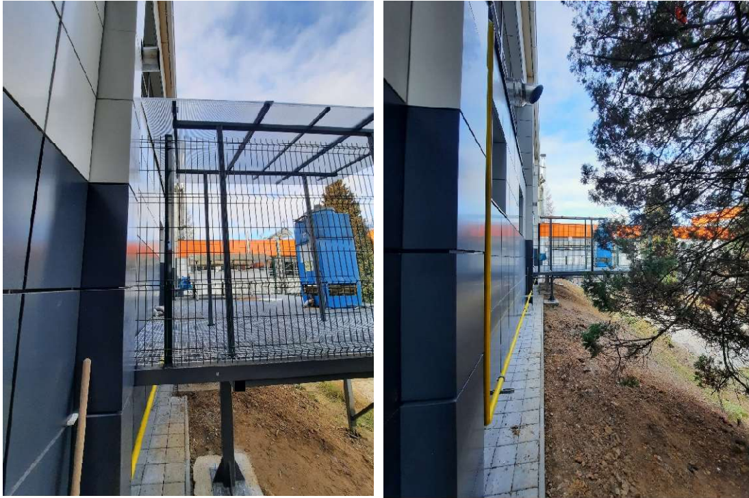
Fig. 8.8 The implemented platform with a shelter prepared for the installation of a small pyrolysis reactor, view of the platform location in the terrain near the laboratory of the Department of Energy Machines and Equipment
