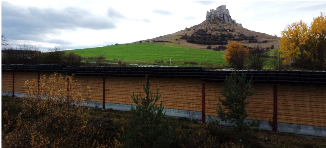
Fig. 3.18 View of the installed noise absorbers in the given section – rear view
