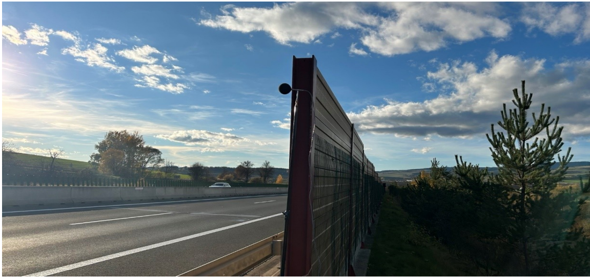
Fig. 3.28 View of measurement point M5
