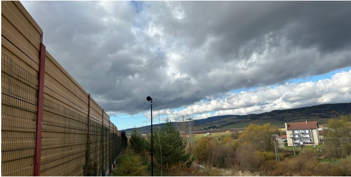
Fig. 3.24 View of measurement point M2
