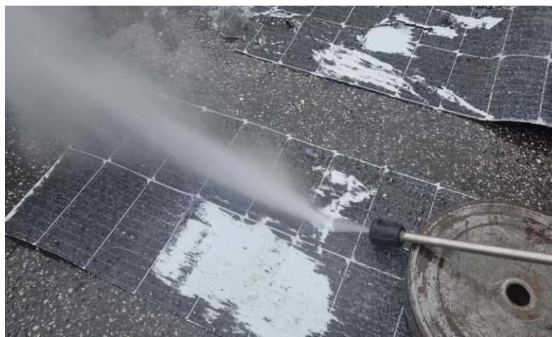
Fig. 1.22 Removing 3 layers with a water jet
