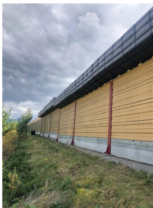
Fig. 3.12 Installed noise absorbers on the noise barrier
