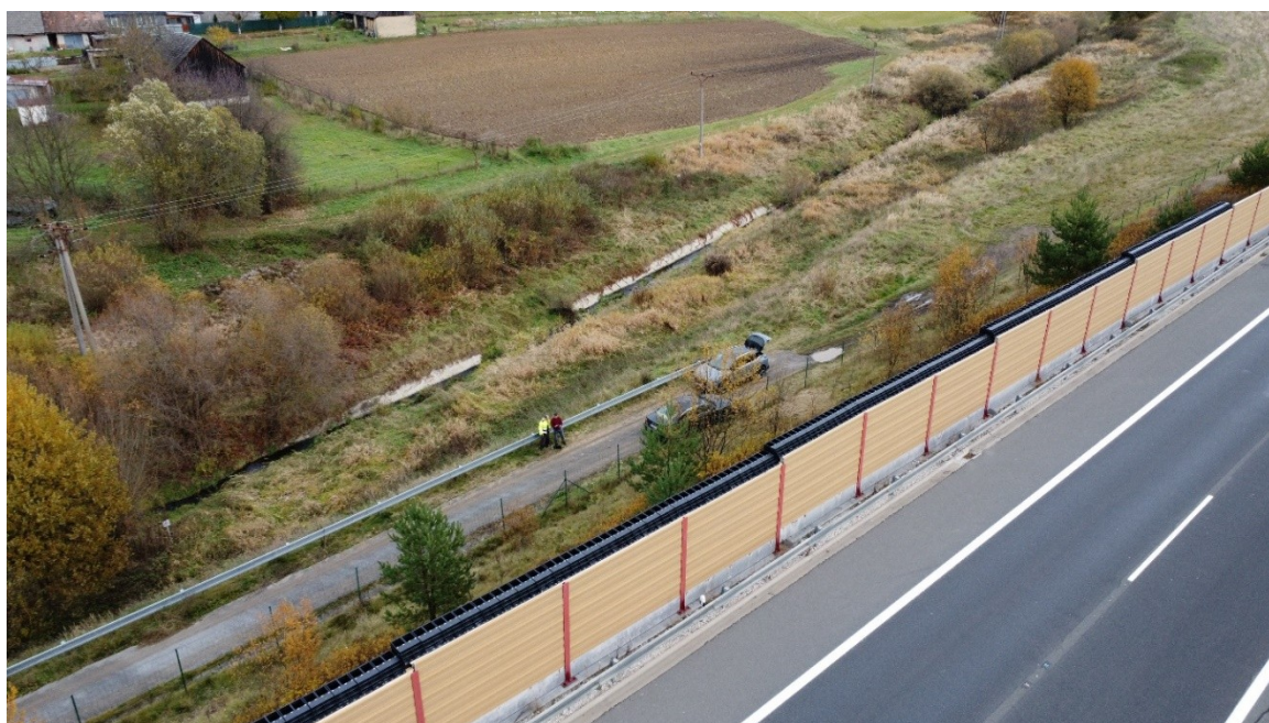
Fig. 3.13 Aerial view of the installed noise absorbers
