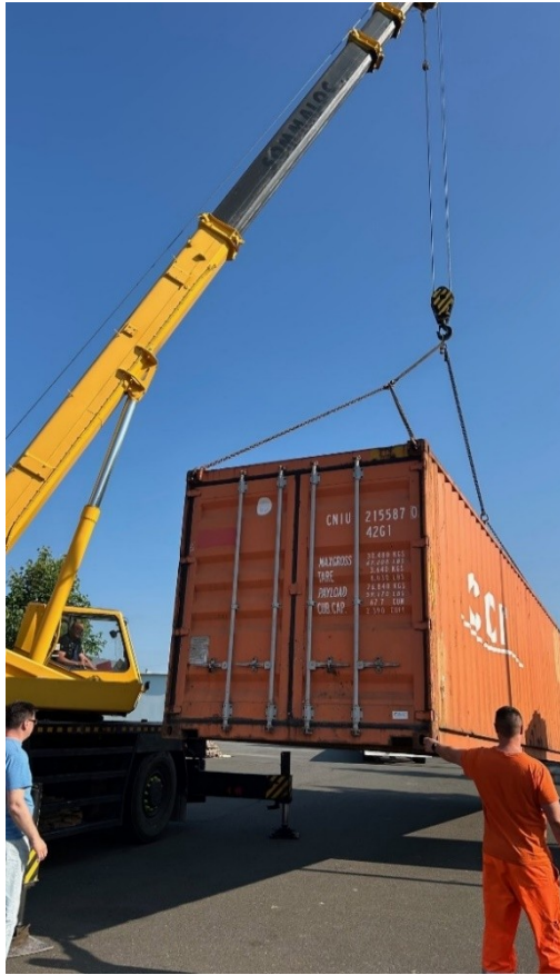
Fig. 3.6 Assembly of the container at the SSÚD Beharovce site
