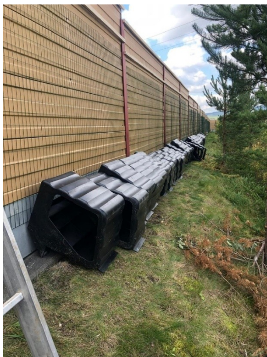
Fig. 3.11 Absorbers prepared for installation
