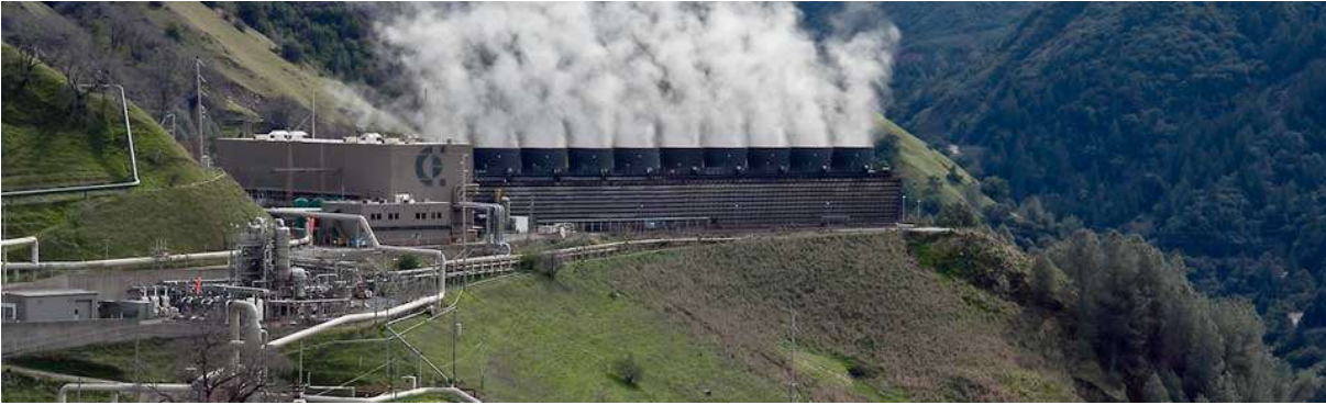
Fig. 76 Geothermal Power Plant in Geysers, USA [94]
