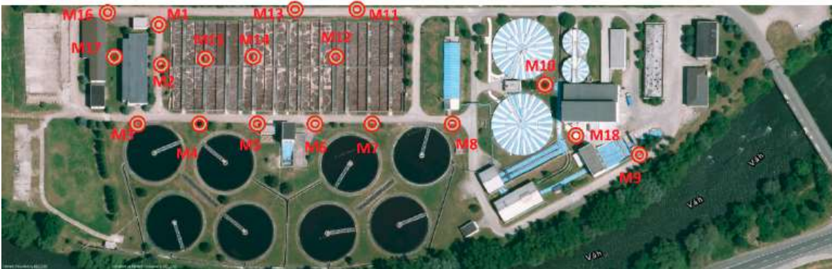
Fig. 235 The locations of the measuring points on the; site of the wastewater treatment plant
