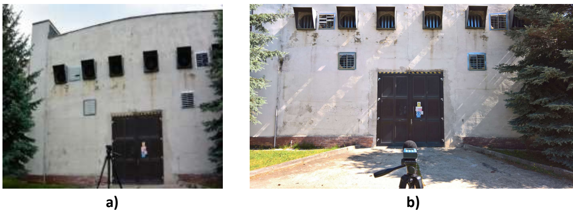
Fig. 250 View of blower room a) before and b) after application measures
