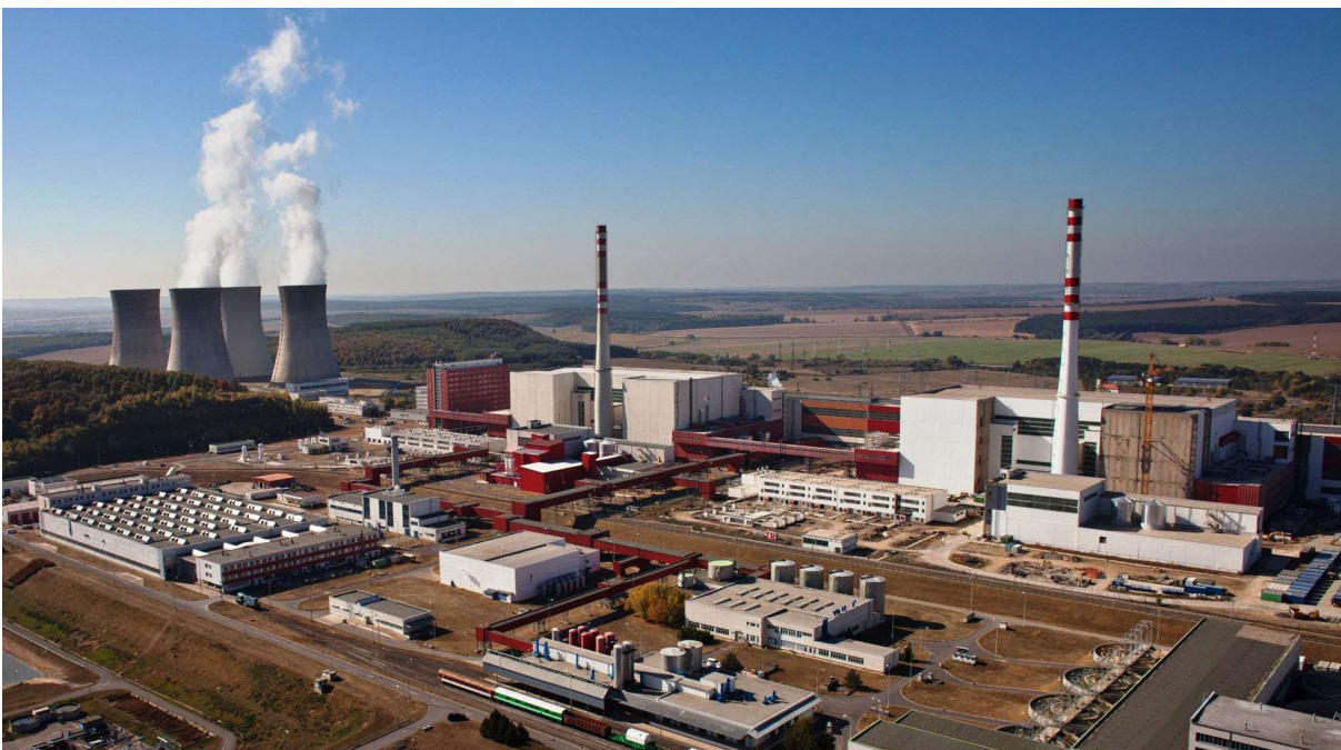
Fig. 33 Nuclear power plant Mochovce [51]
