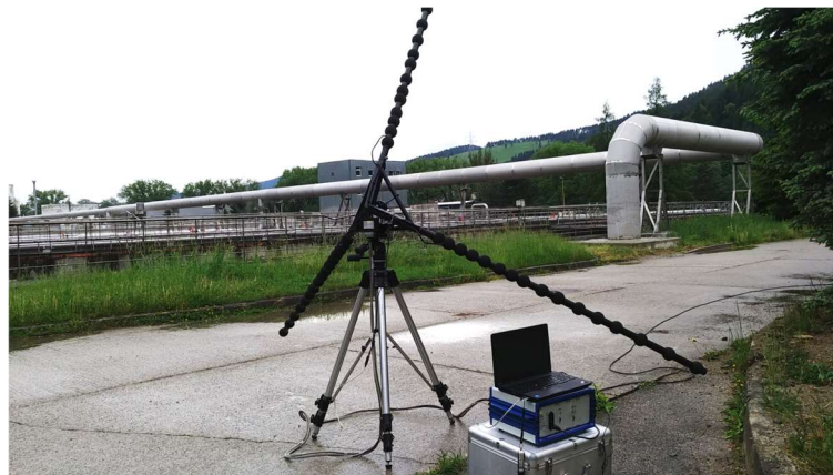
Fig. 236 View of the installed acoustic camera - measurement No. 1.
