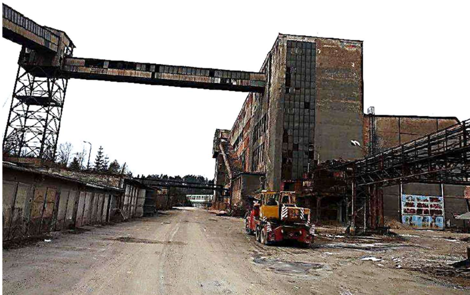
Fig. 265 View of processing plant 2 [186]
