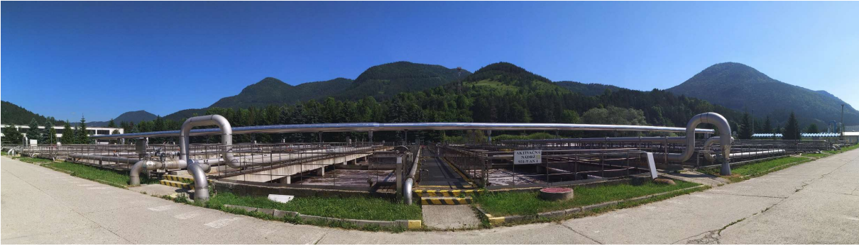
Fig. 232 A view of the treatment plant
