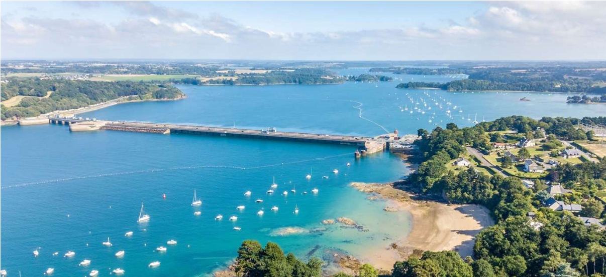
Fig. 71 Tidal hydroelectric power plant in the estuary of the French River La Rance [89]
