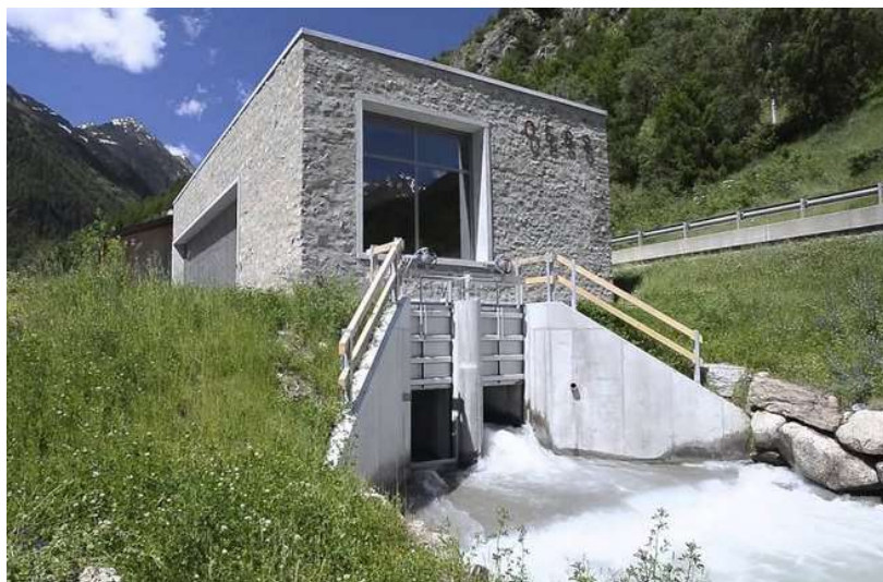
Fig. 53 Small hydroelectric power plant [78]
