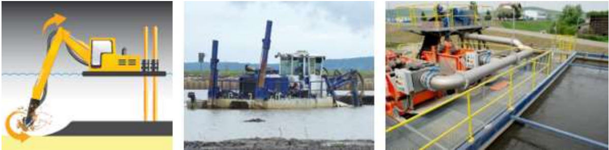
Fig. 143 Remediation operations at the bottom of the tank [120]
